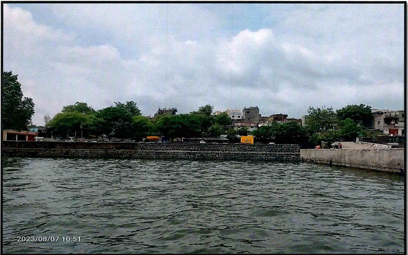
South Bank Part 1 after Restoration
