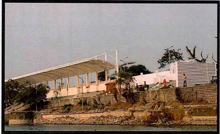
East Bank in dilapidated condition
