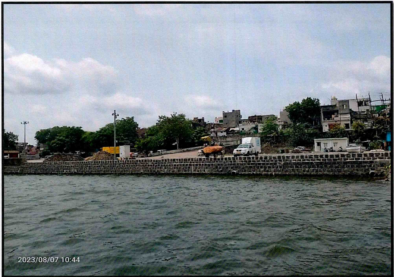
South Bank Part 2 after Restoration
